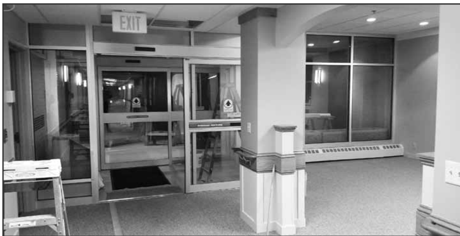
Pictured, ABOVE and to the RIGHT: The new renovation of the entrance and lobby area of the D.J. Jacobetti Home will be completed within the next week or so. Home Administrator Brad Slagle and Home Maintenance Manager Mike Harrington have worked tirelessly to get these renovations completed.
